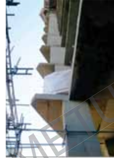
Walking Columns: Better alternative than bulky transfer slabs or beams [1]
